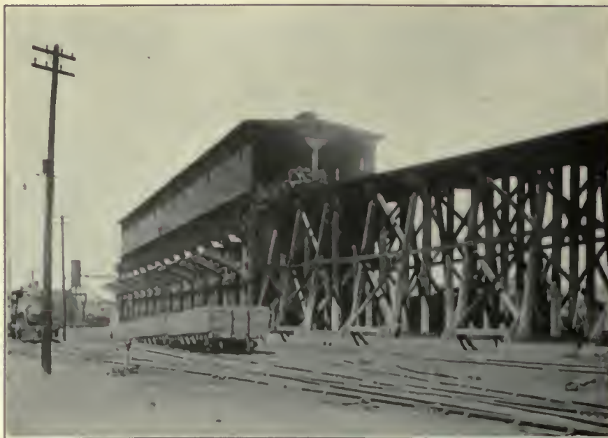
FIG. 665. FACILITIES TO BE ABANDONED. Wooden coaling station of the Chicago & North Western Railway, near N. Karlov and Austin avenues. This station was built in 1902 at an approximate cost of $50,000 and has a storage capacity of 1,600 tons of coal. In the event of electrification, this structure will be rendered worthless.
